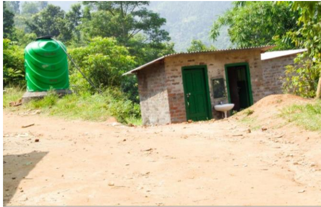
Fig: Installation of water facility in front of the toilet
