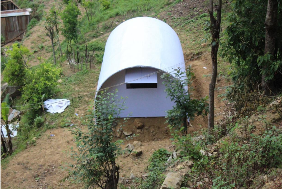
Fig: A shelter prototype installed at the place
