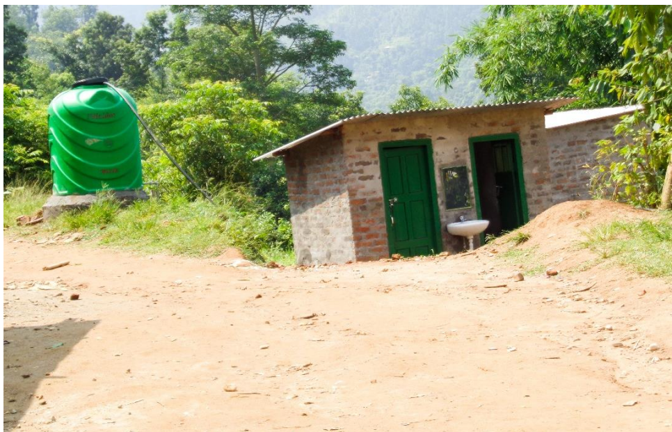
Fig 4. Water and Sanitation Construction
