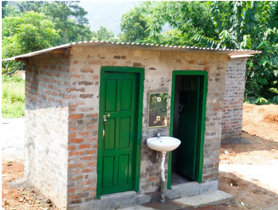
Fig 1. Boys Toilet with Washing Facility
