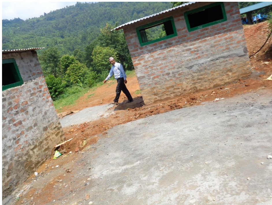
Fig 2. Girls Toilet (Right side) with Safety tank at the front
