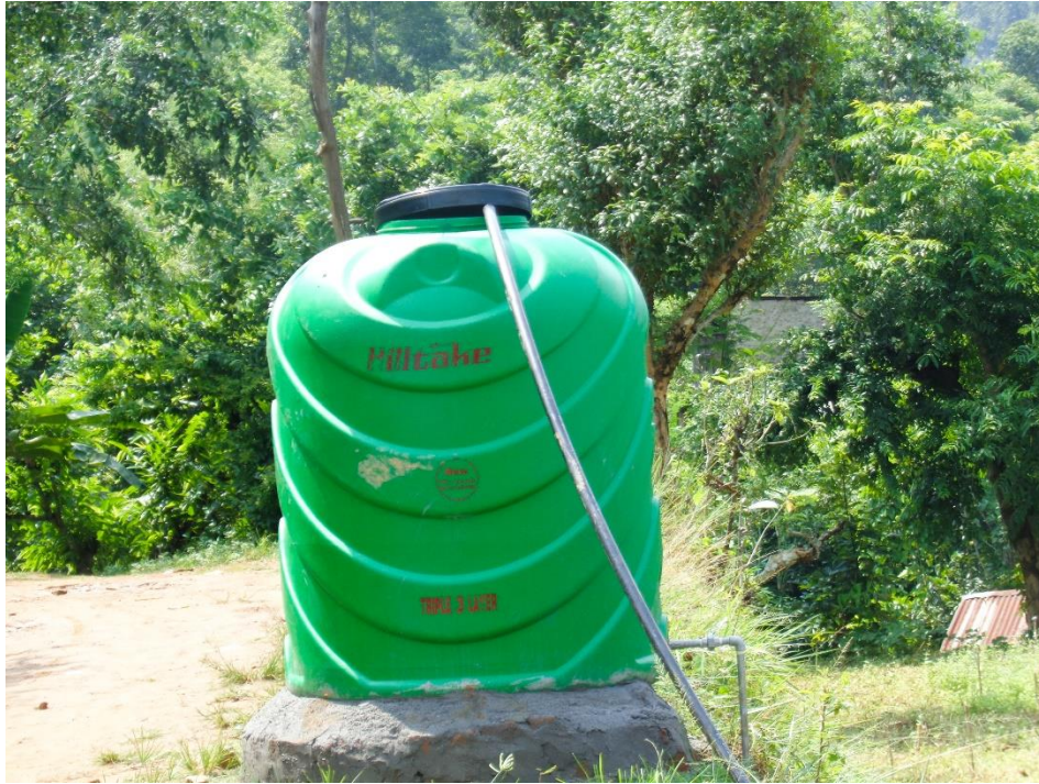
Fig 3. Installation of Water Facility in front of the toilet
