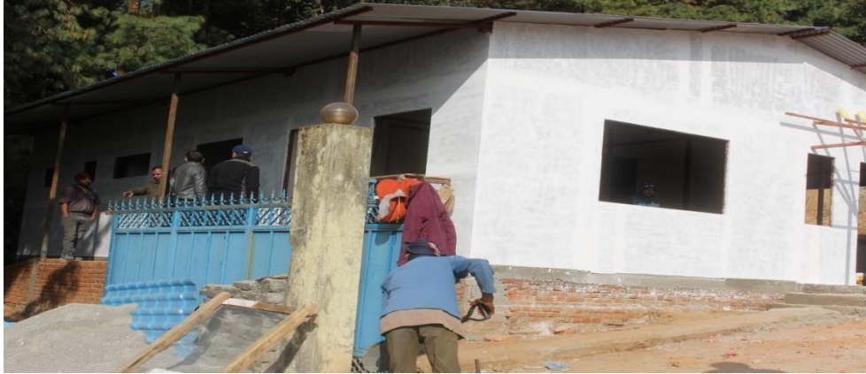
3. Health Post at Tauthali under construction.
