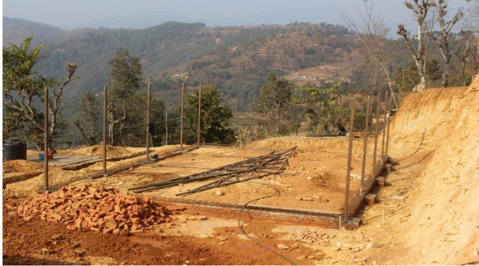
4. Bhotsipa Health Post under construction.
