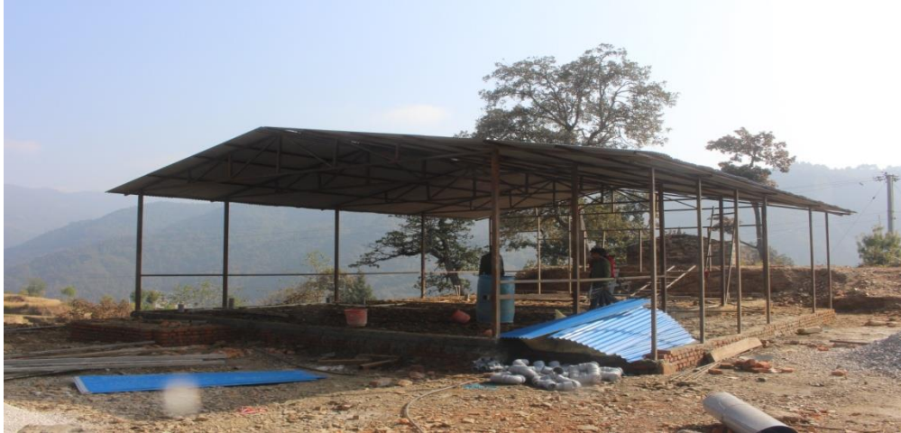
5. Attarpur Healthpost Under Construction.
