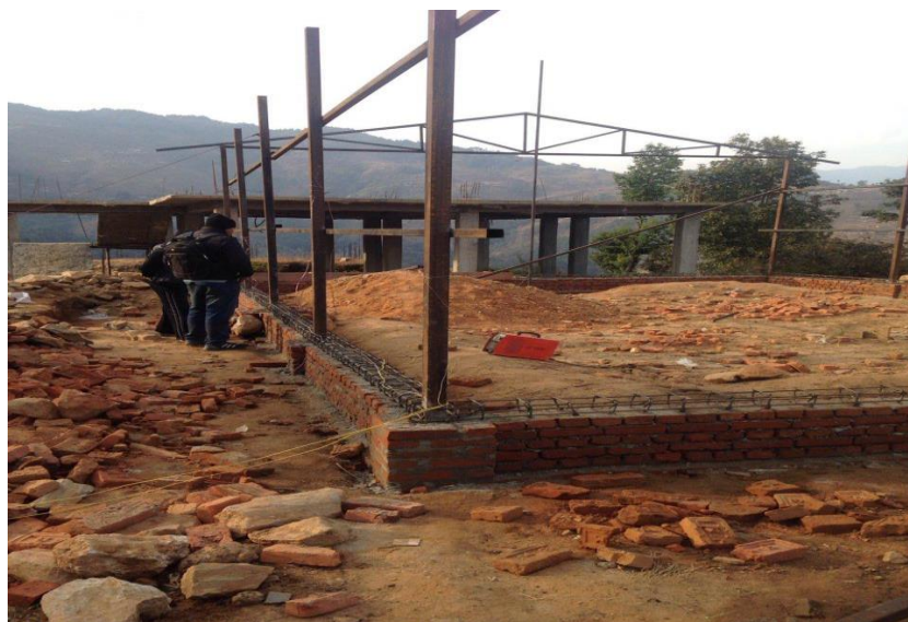
6. Haibung Health post Under Construction
