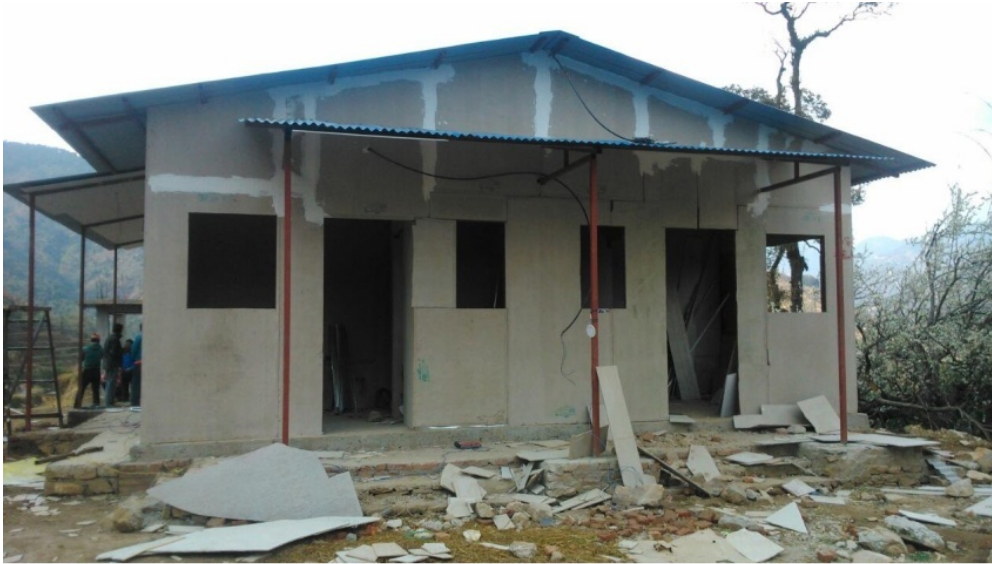
Wall Installation and Finishing work ongoing at Haibung HP
