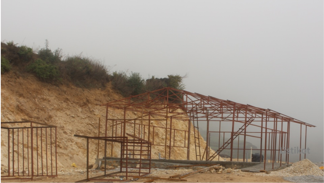
Listikot Helthpost Reconstruction after truss installation.
