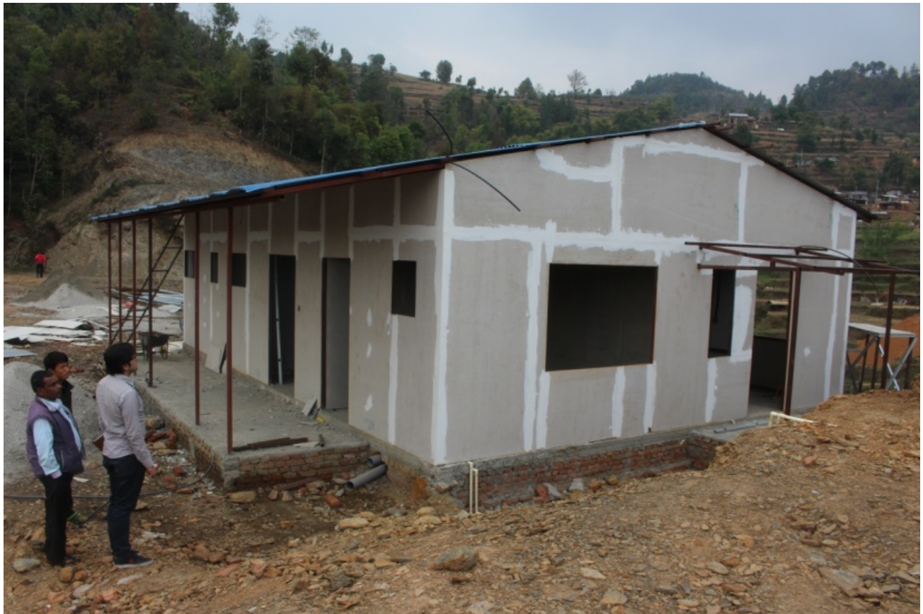
Attarpur Health Post: Wall installation and finishing work ongoing.
