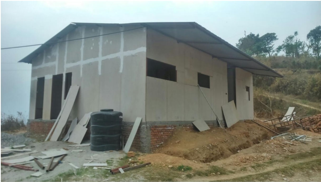
Ongoing Construction at Sipapokhare: Wall insatllation and finishing work
