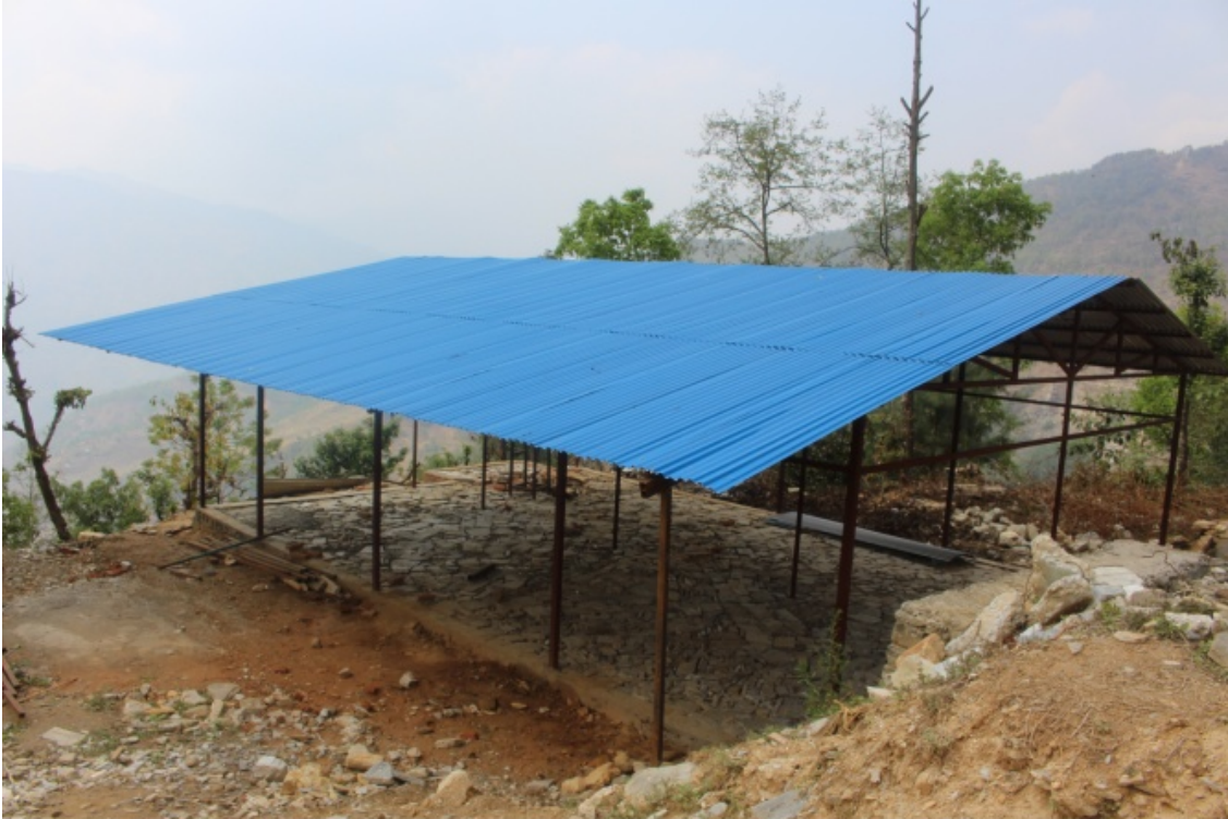
Piskar Health post after completion of Truss work.
