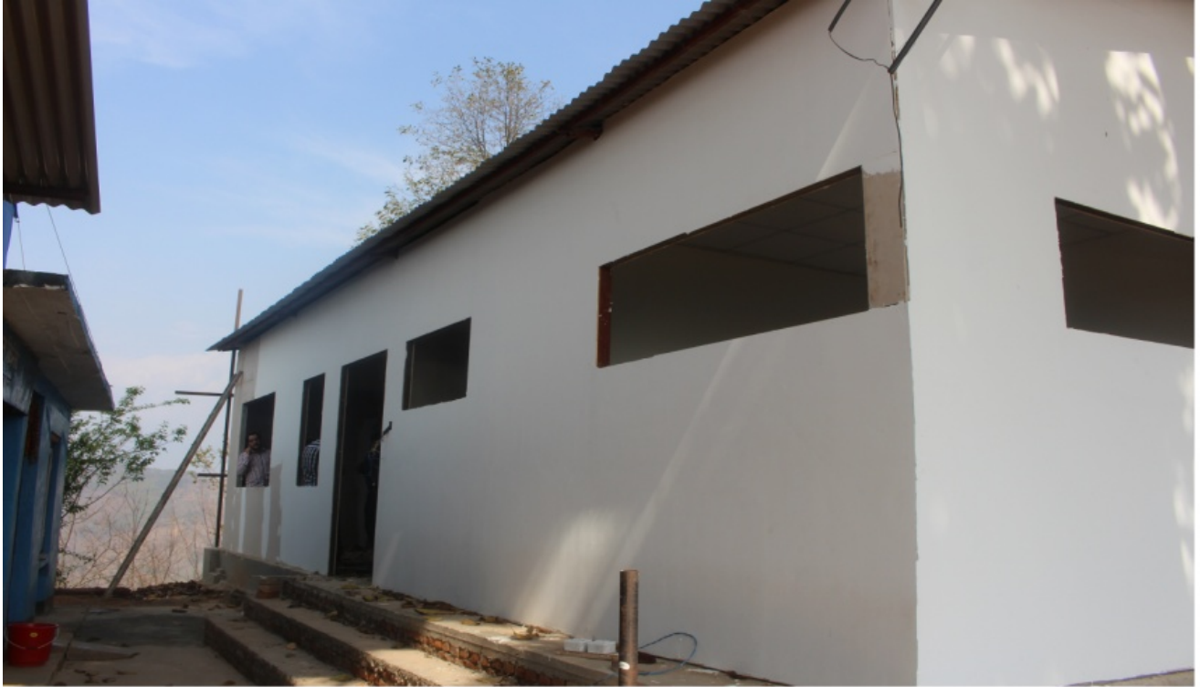
Ongoing Painting and Finishing work at Thulosirubari
