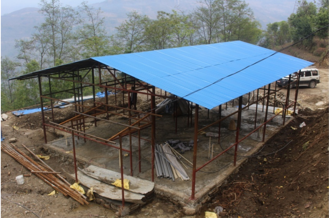
Truss work and Wall framing at Petku
