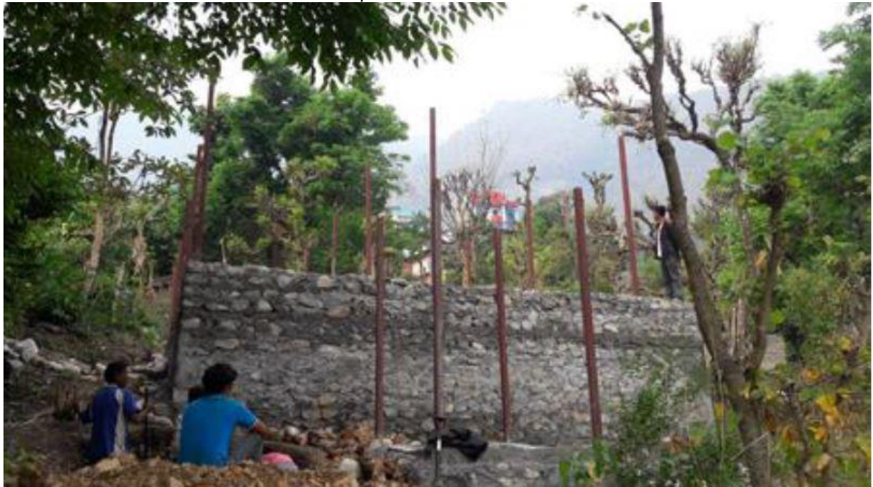
Toilet and septic foundation
