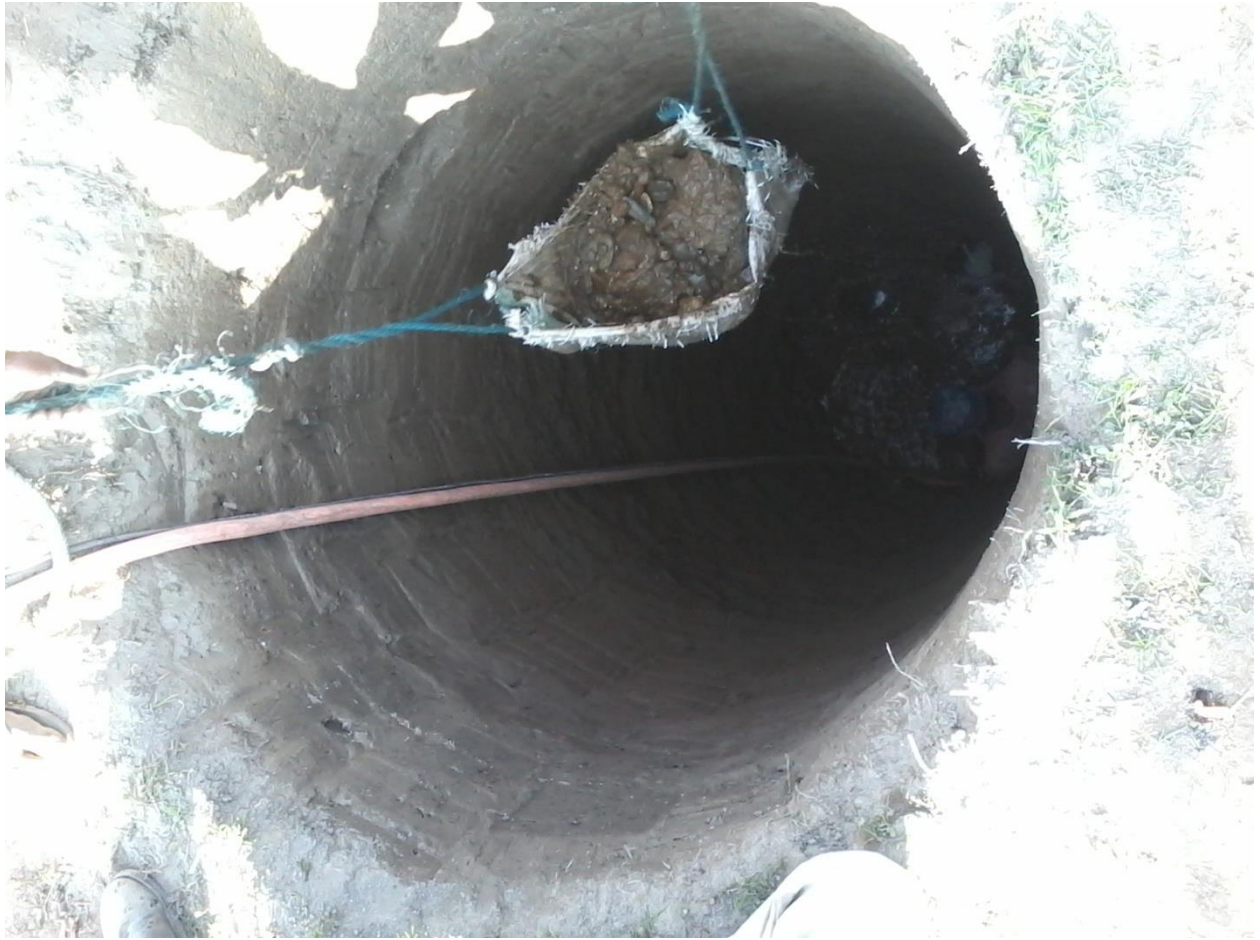
Constructing a well
