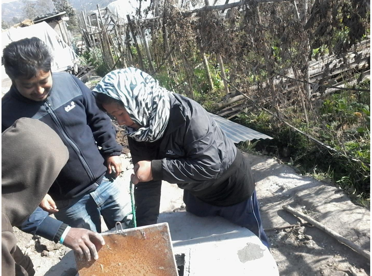
Newly built well
