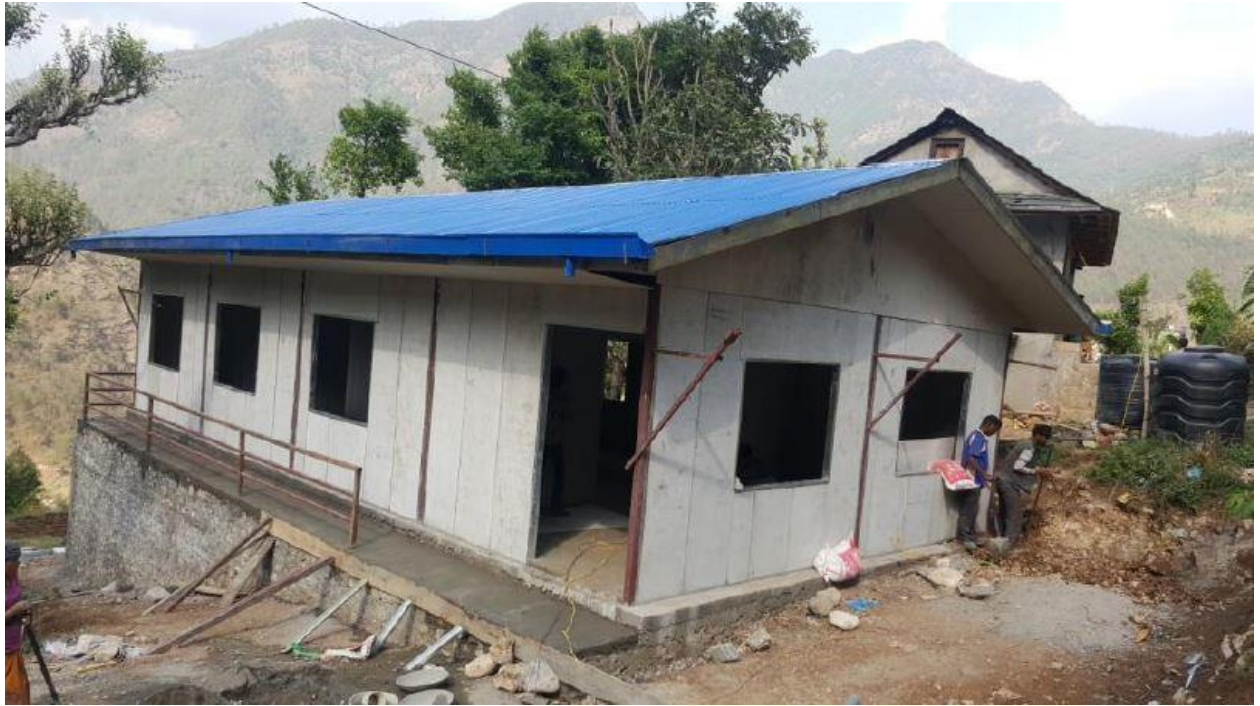
CGI sheet installation
