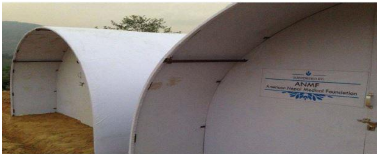
Health post and birthing centre at Talakhu, Nuwakot
