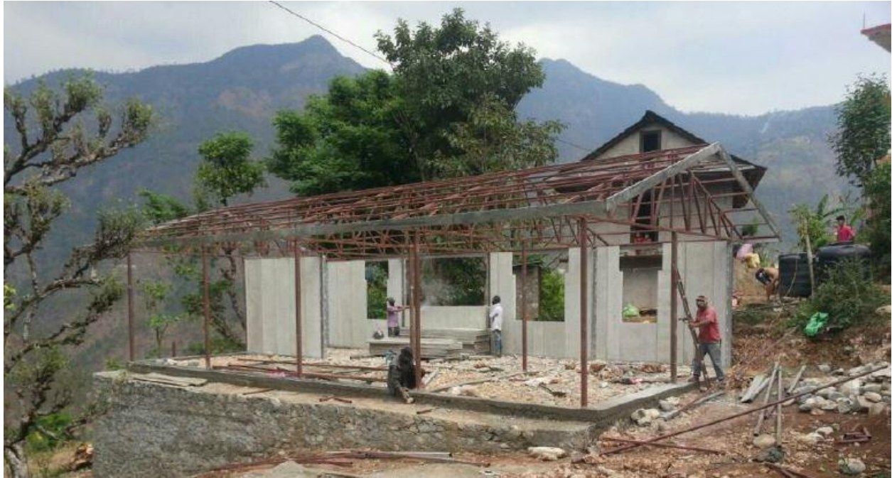
Prefab board installation
