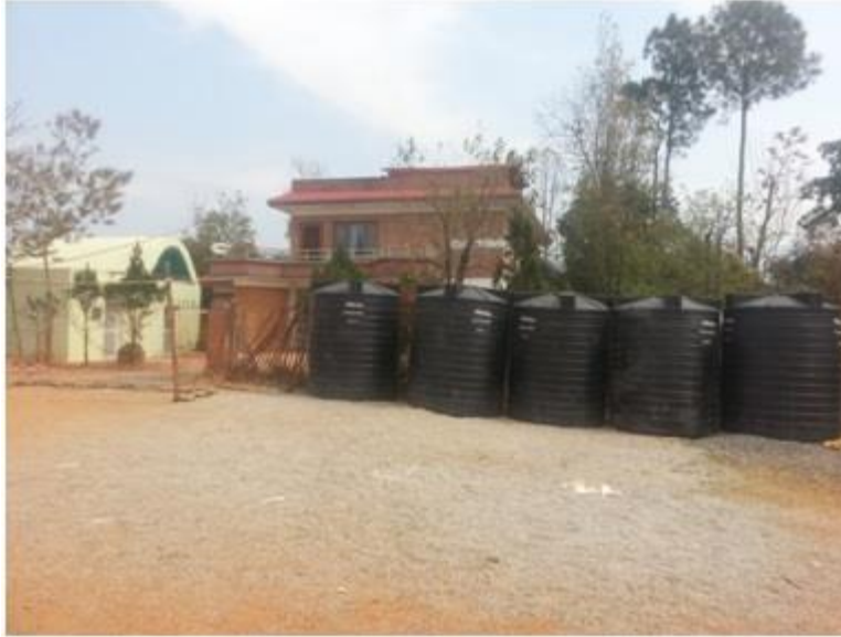
Water tanks at Baruwa
