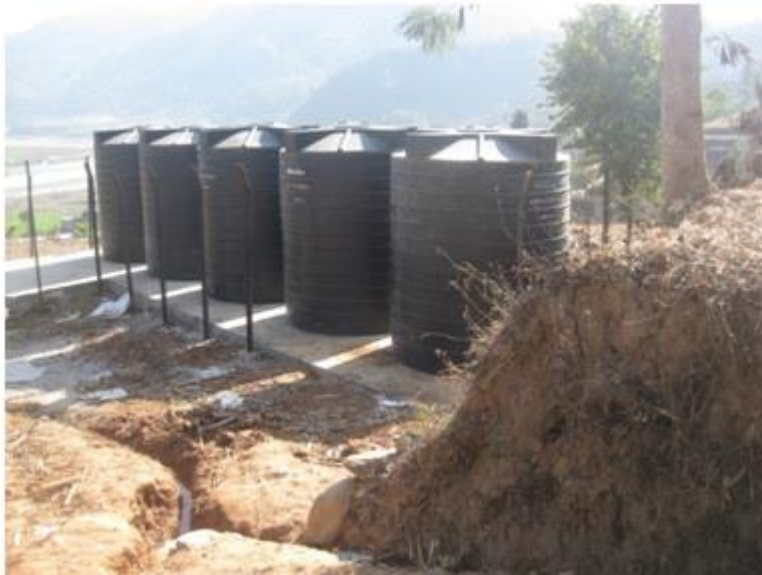
Water tank installed at Bahunepati
