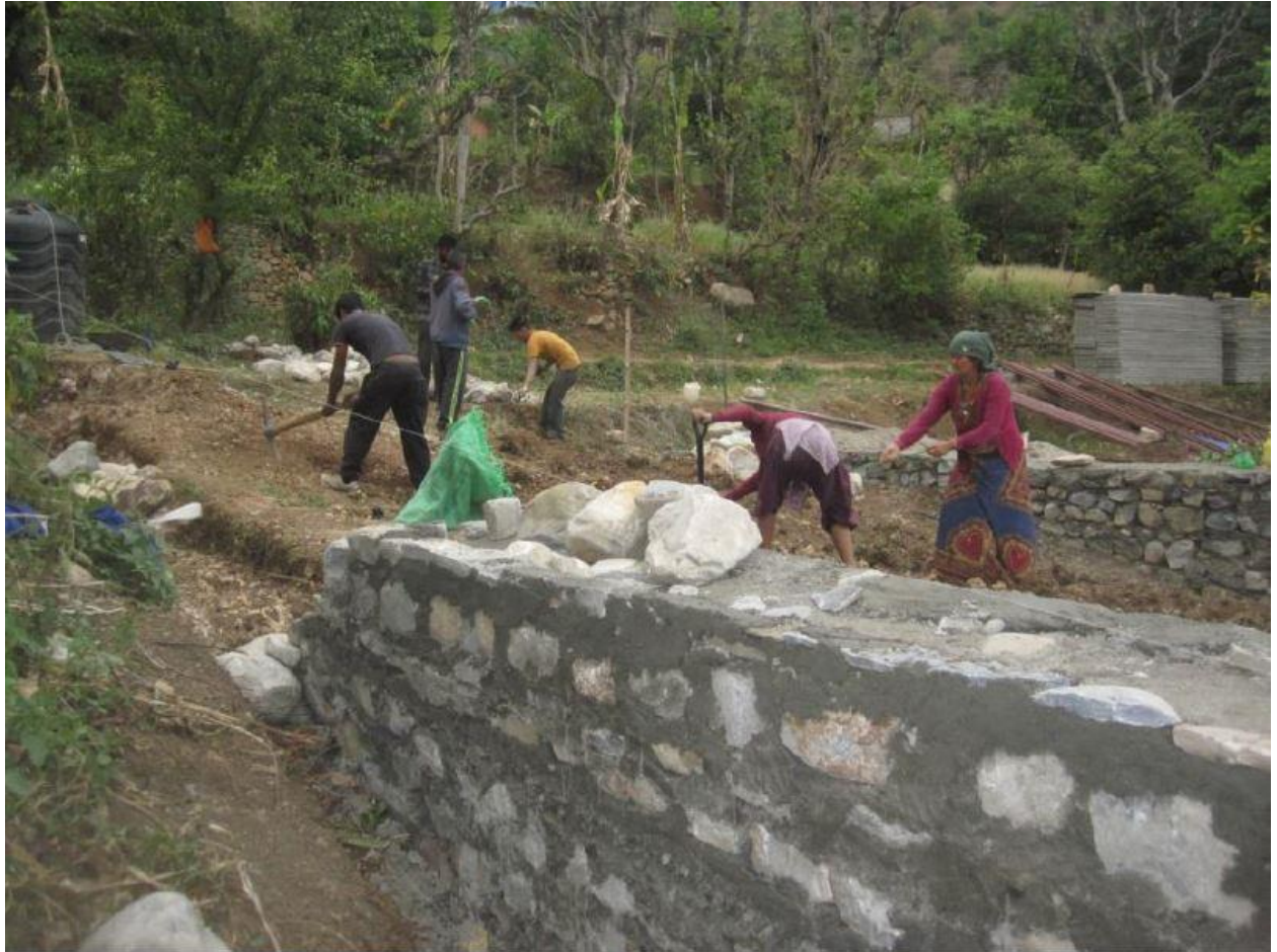
Excavation for leveling and filling
