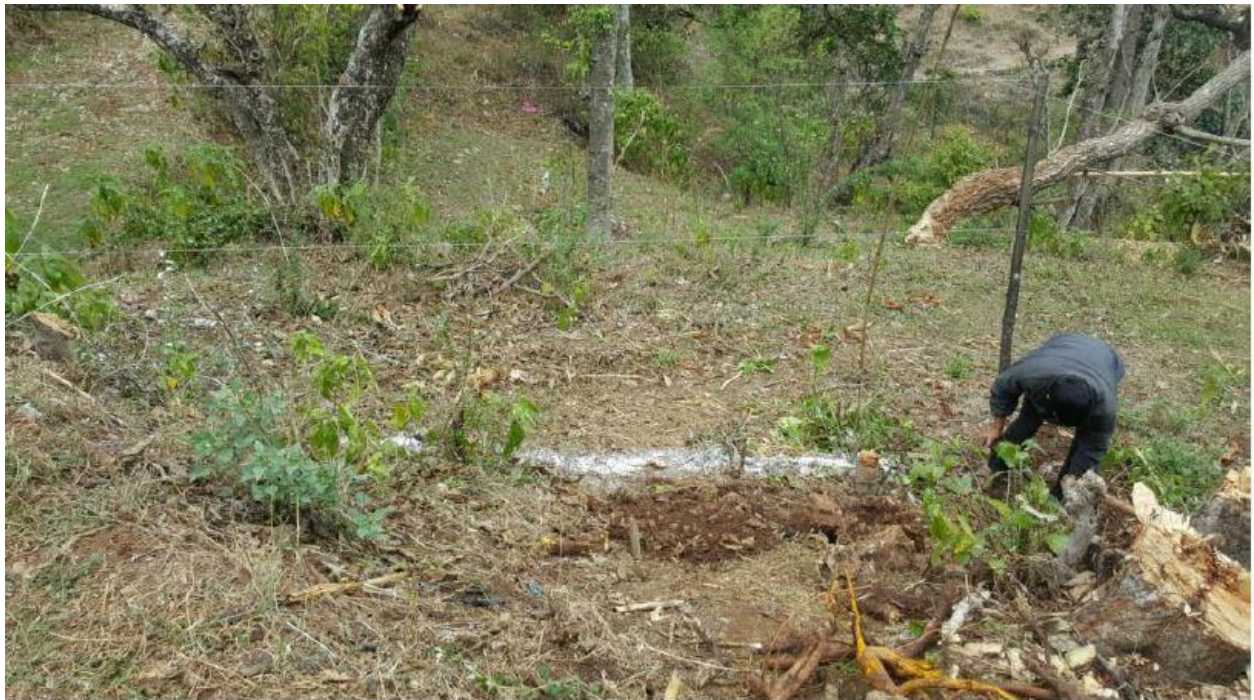
Land layout and site clearance
