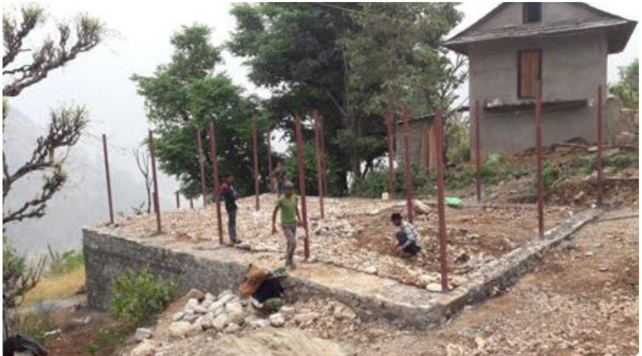
Leveling and flooring (Foundation work)
