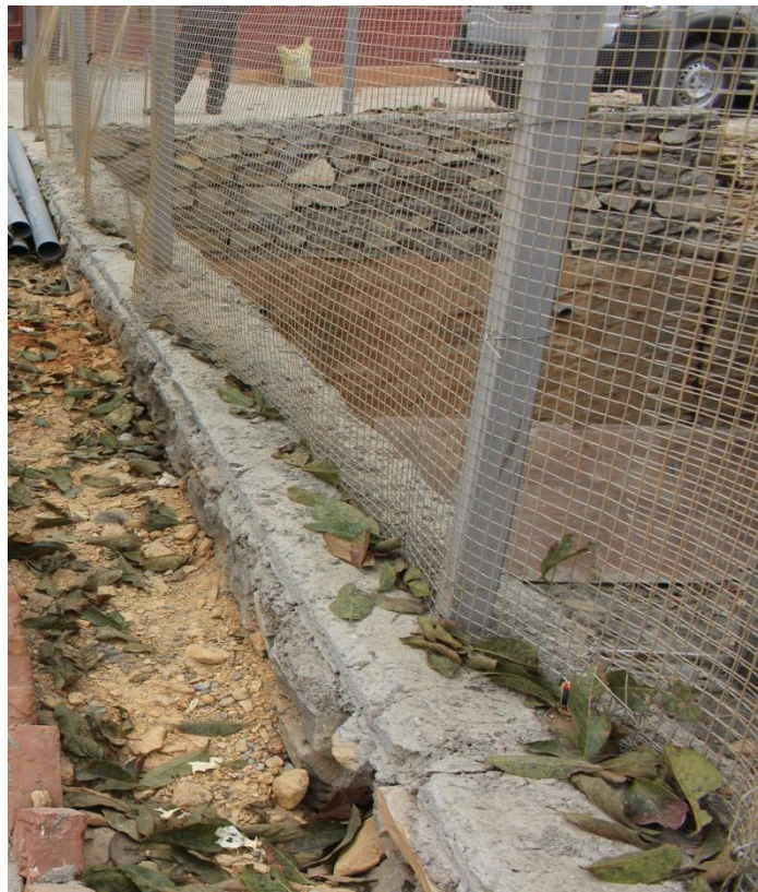
A retaining wall and a net constructed besides the prefabricated structure
