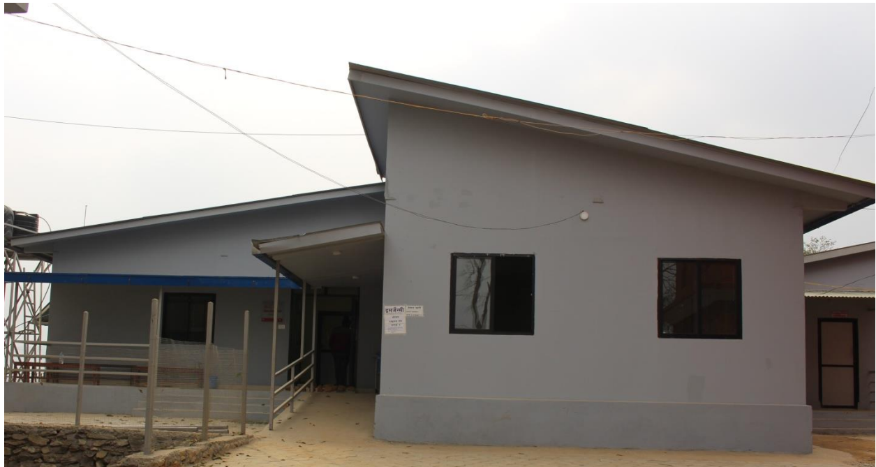
Chautara prefabricated structure
